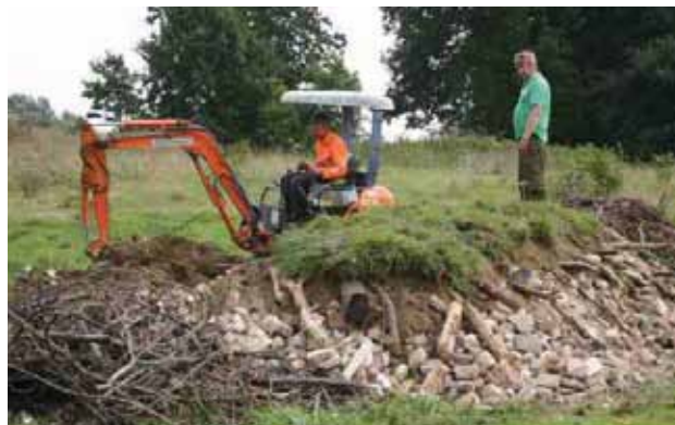
A reptile bank under construction. Turf has been stripped to create a shallow pit to receive a pile of hardcore and logs. This will be covered with the stripped turves (Lee Brady)
